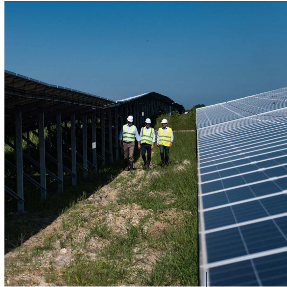
DURING CONSTRUCTION OF THE SOLAR PARK PARADISE PARK, JAMAICA
